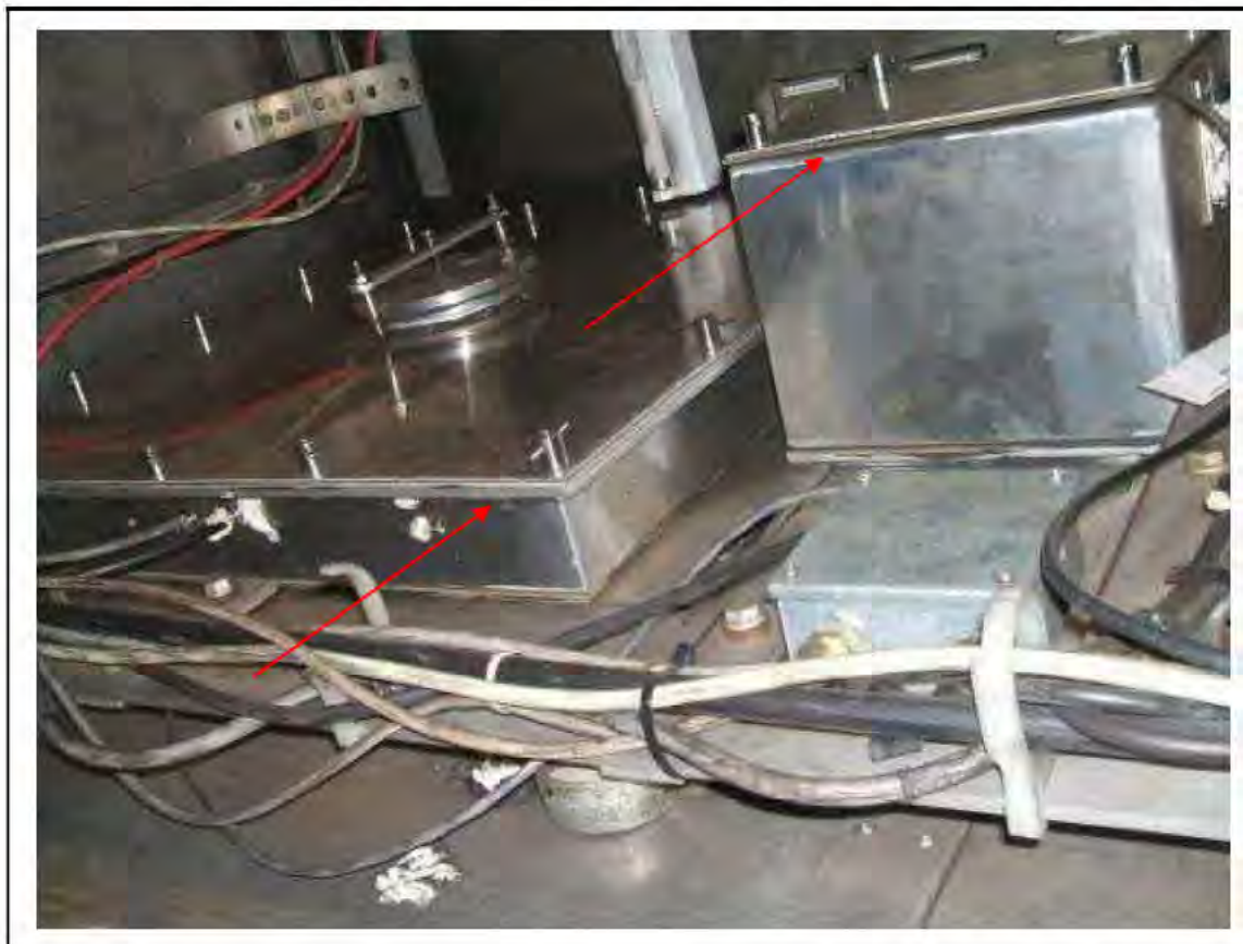
FIGURE 160: STRONGLY PRESUMED ASBESTOS IN POSSIBLE SILUMINITE PACKING IN IMR (CORRIDOR TO PLATFORM 2), 3/706 - DESCRIPTION & RESULT OF ASSESSMENT (SAMPLE REF. SP1(12))
