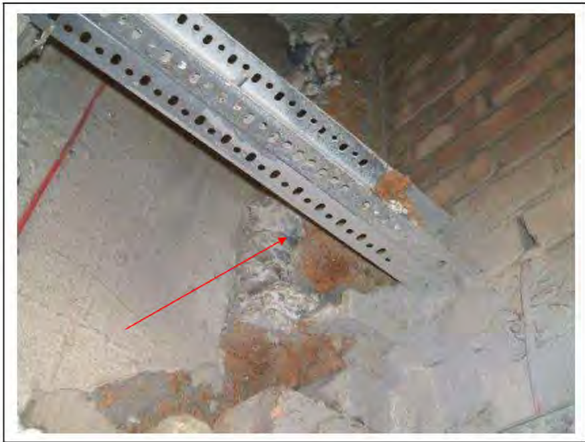
FIGURE 41: PRESUMED ASBESTOS IN RESIDUE BEHIND FOAM SEAL IN PASSAGE , 2/238 - DESCRIPTION & RESULT OF ASSESSMENT (SAMPLE REF. P1&2(28))
