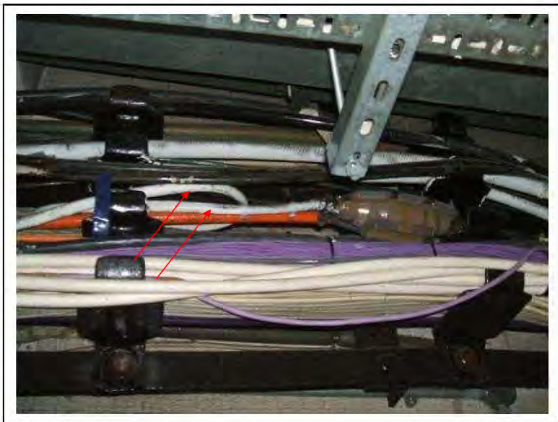
FIGURE 26: KNOWN ASBESTOS IN BRAIDED CABLES IN UMC, 2/151 - DESCRIPTION & RESULT OF ASSESSMENT (SAMPLE REF. K1(3))
