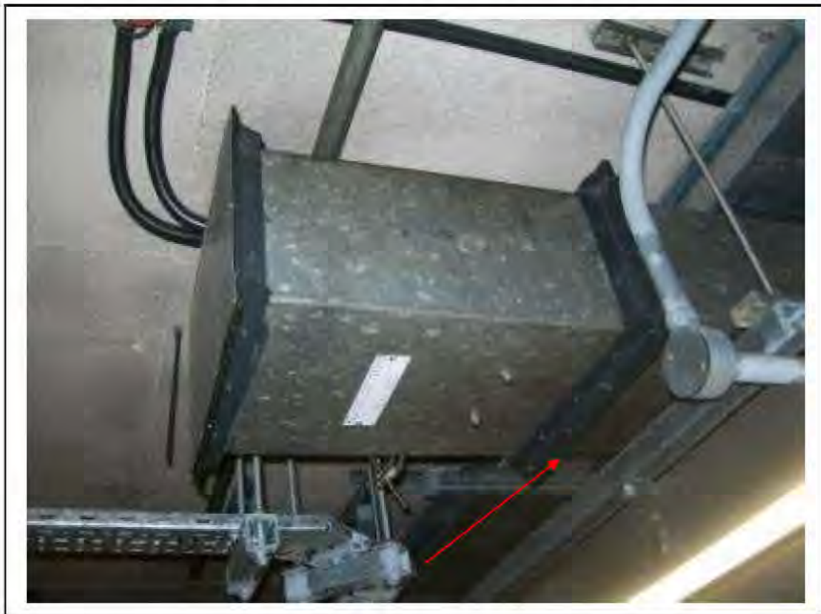
FIGURE 30: KNOWN ASBESTOS IN GASKET IN UMC , 2/151 - DESCRIPTION & RESULT OF ASSESSMENT (SAMPLE REF. K1(4))
