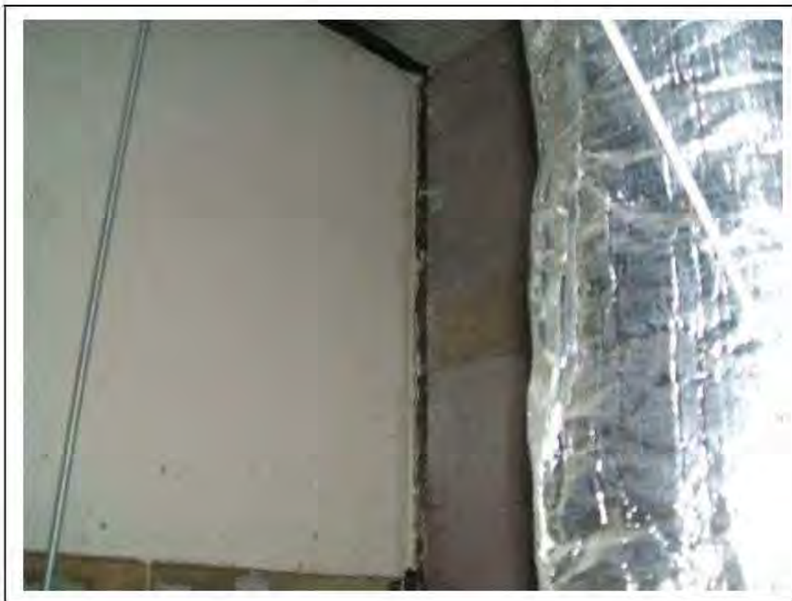
FIGURE 56: PRESUMED ASBESTOS IN RESIDUES IN MALE W/C, 2/417 - DESCRIPTION & RESULT OF ASSESSMENT (SAMPLE REF. P1&2(42))
