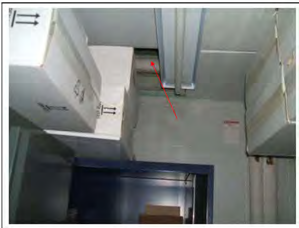
FIGURE 51: PRESUMED ASBESTOS IN RESIDUES TO CAVITY IN STORE , 2/413 - DESCRIPTION & RESULT OF ASSESSMENT (SAMPLE REF. P1&2(37))
