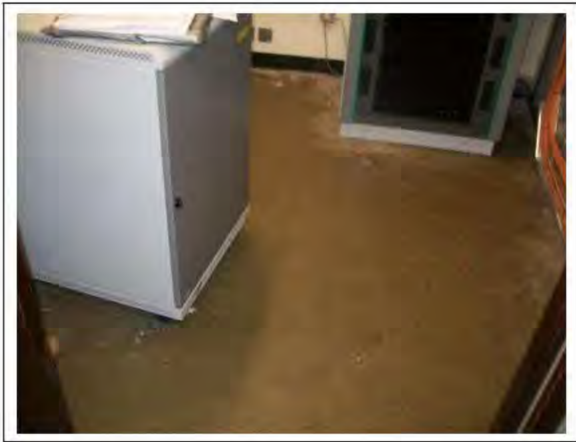
FIGURE 144: CONFIRMED ASBESTOS IN MARLEY TILES ON CONCRETE SLAB IN CER (OLD), 3/668 - DESCRIPTION & RESULT OF ASSESSMENT (SAMPLE REF. 120445/150812/01)
