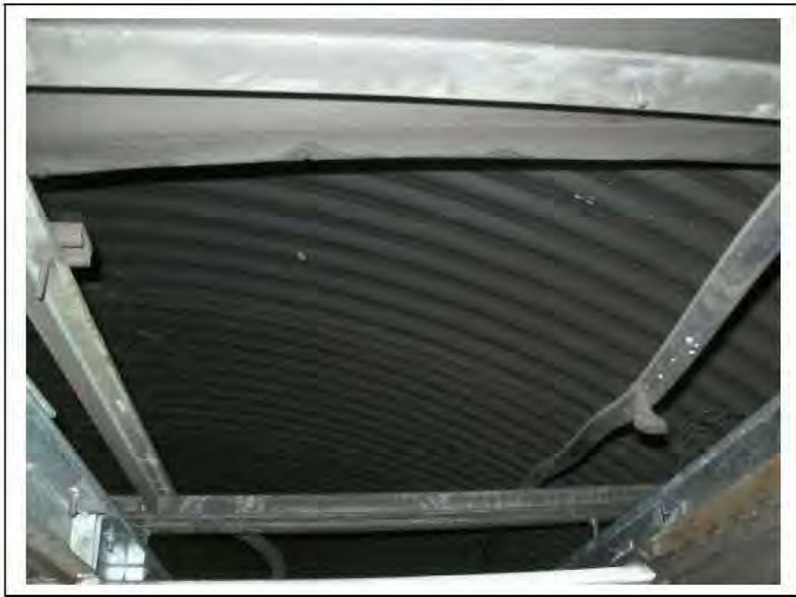
FIGURE 100: KNOWN ASBESTOS IN CELLACTITE IN PASSAGE , 3/209 - DESCRIPTION & RESULT OF ASSESSMENT (SAMPLE REF. K1(23))
