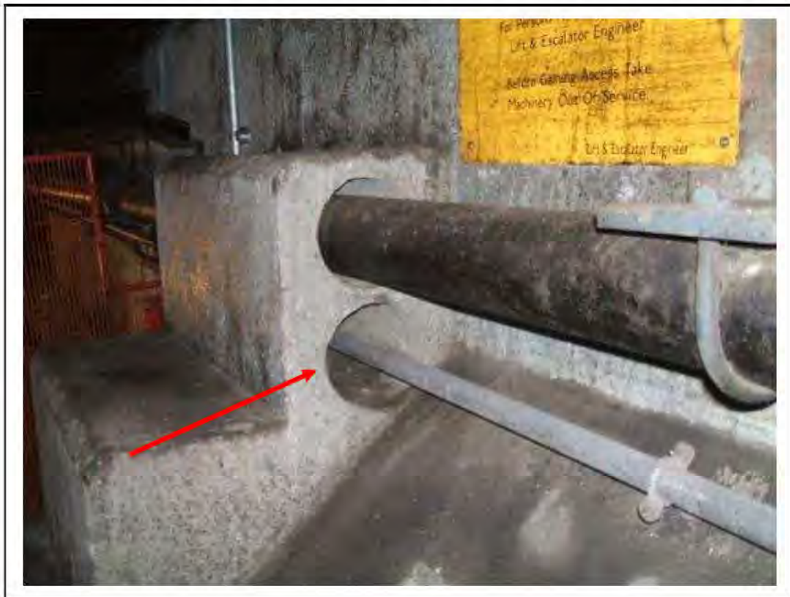
FIGURE 80: CONFIRMED ASBESTOS IN DUCTS IN LMC, 3/161 - DESCRIPTION & RESULT OF ASSESSMENT (SAMPLE REF. 120445/130812/1)
