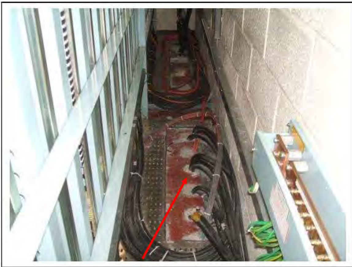
FIGURE 133: PRESUMED ASBESTOS IN DUCTS IN SER, 3/371 - DESCRIPTION & RESULT OF ASSESSMENT (SAMPLE REF. P1(9))
