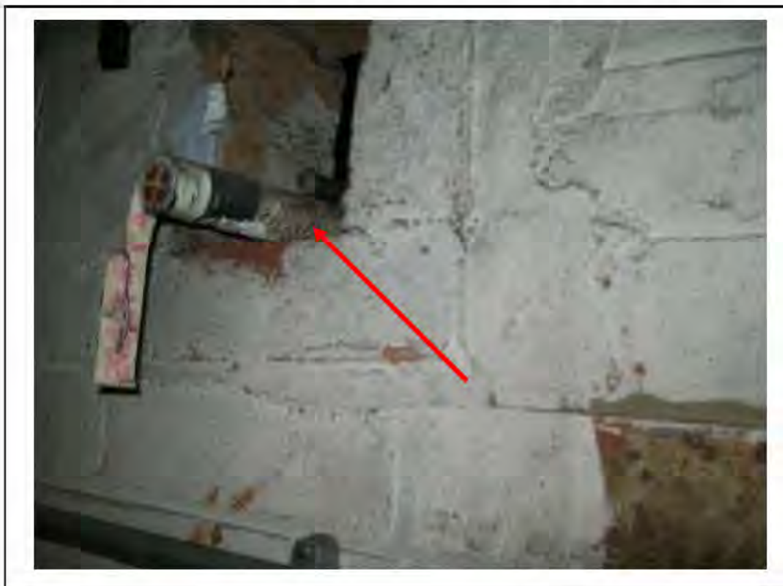
FIGURE 31: KNOWN ASBESTOS IN CABLE BRAIDED IN UMC , 2/151 - DESCRIPTION & RESULT OF ASSESSMENT (SAMPLE REF. K1(5))
