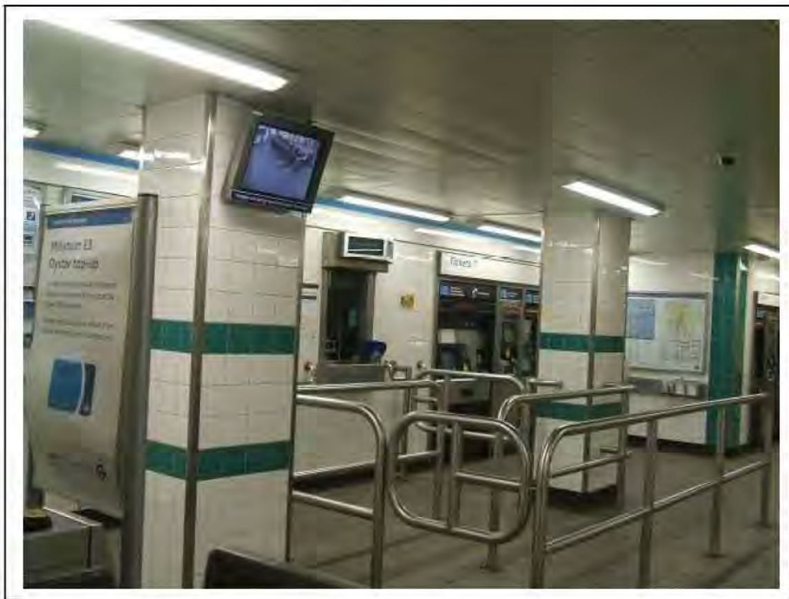
FIGURE 10: PRESUMED ASBESTOS ABOVE FALSE CEILING IN CIRCULATION AREA, 2/071 - DESCRIPTION & RESULT OF ASSESSMENT (SAMPLE REF. P1&2(10))
