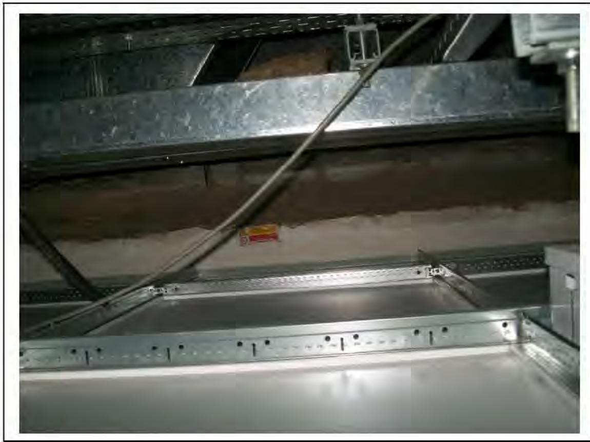
FIGURE 6: PRESUMED ASBESTOS IN RESIDUAL SPRAY INSULATION WITHIN CAVITY IN POM, 2/021 - DESCRIPTION & RESULT OF ASSESSMENT (SAMPLE REF. P1&2(6))
