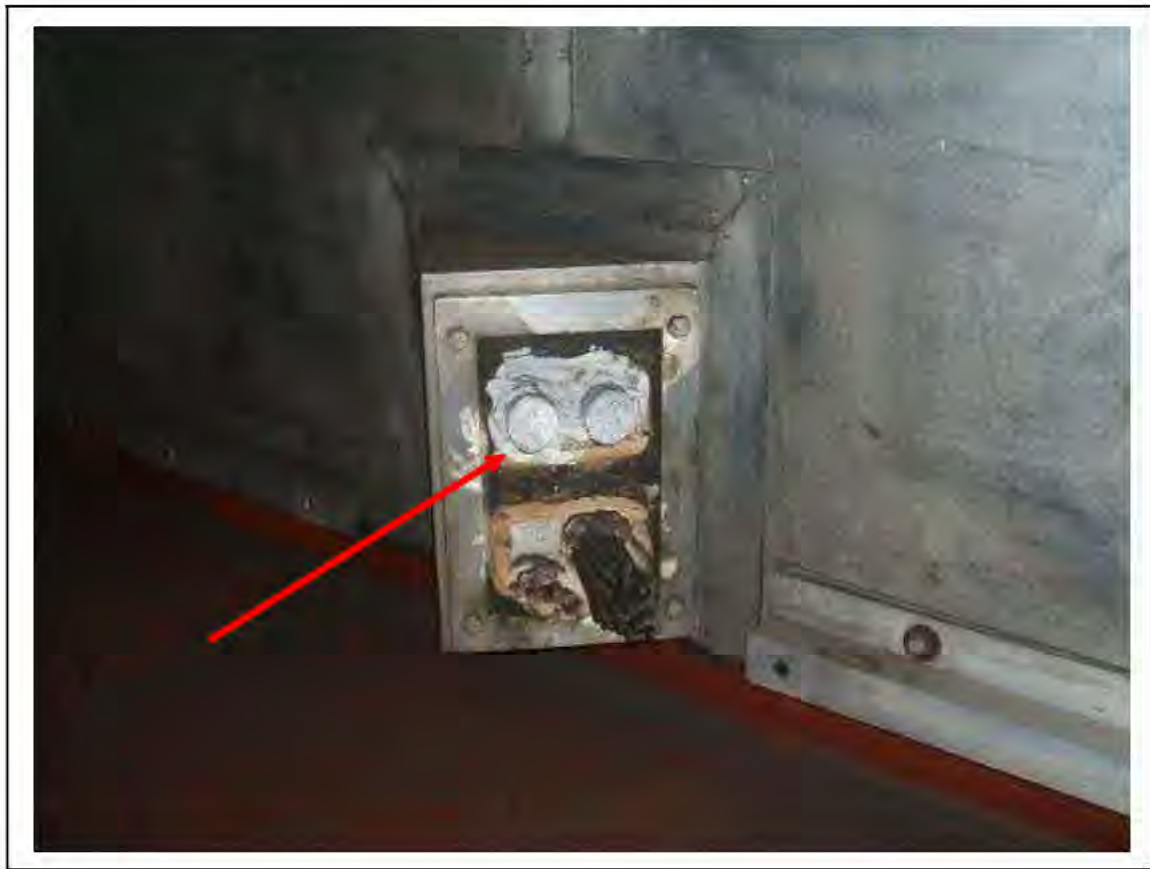
FIGURE 162: KNOWN ASBESTOS IN BRAIDED CABLE IN IMR, 3/707 - DESCRIPTION & RESULT OF ASSESSMENT (SAMPLE REF. K1(42))
