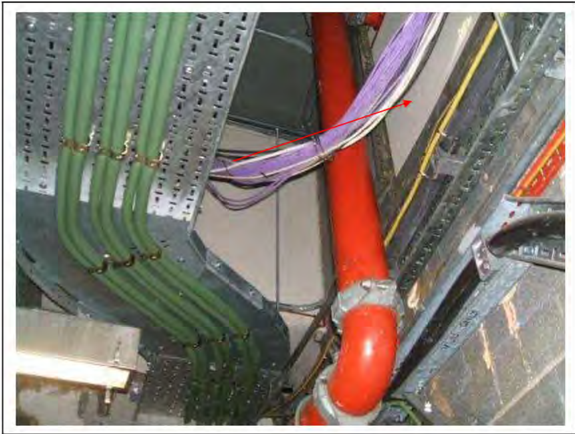
FIGURE 12: PRESUMED ASBESTOS IN SUPALUX PANEL IN UMC ACCESS , 2/151 - DESCRIPTION & RESULT OF ASSESSMENT (SAMPLE REF. P1&2(12))
