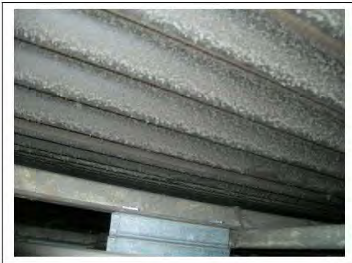
FIGURE 93: KNOWN ASBESTOS IN CELLACTITE IN PASSAGE, 3/206 - DESCRIPTION & RESULT OF ASSESSMENT (SAMPLE REF. K1(18))
