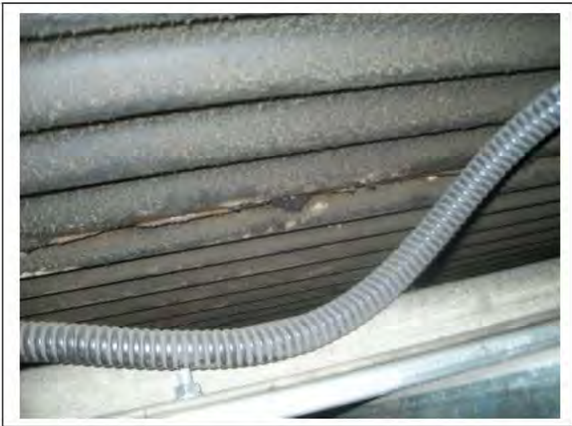
FIGURE 84: KNOWN ASBESTOS IN CELLACTITE IN PASSAGE , 3/201 - DESCRIPTION & RESULT OF ASSESSMENT (SAMPLE REF. K1(13))
