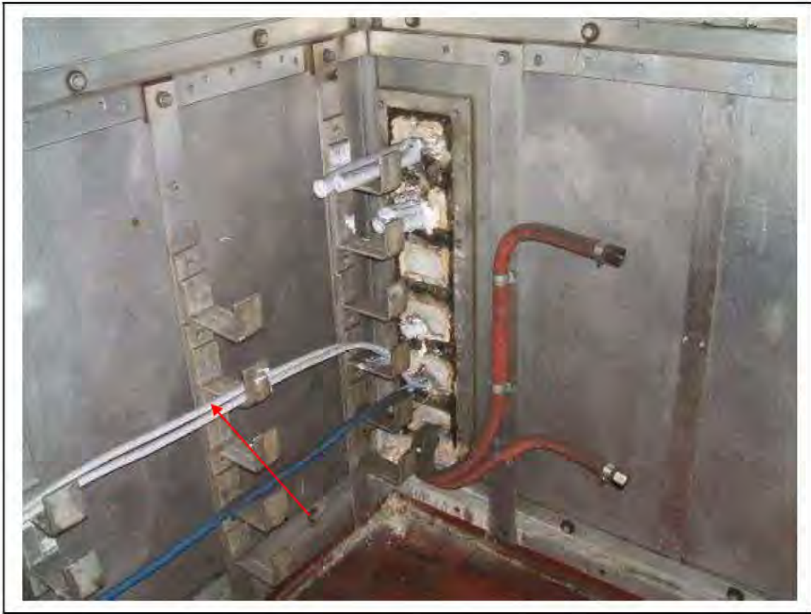
FIGURE 153: KNOWN ASBESTOS IN BRAIDED CABLES IN IMR, 3/706 - DESCRIPTION & RESULT OF ASSESSMENT (SAMPLE REF. K1(37))
