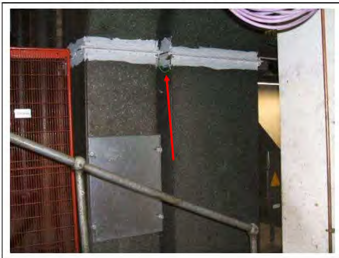
FIGURE 20: KNOWN ASBESTOS IN GASKETS IN UMC, 2/151 - DESCRIPTION & RESULT OF ASSESSMENT (SAMPLE REF. K1(1))
