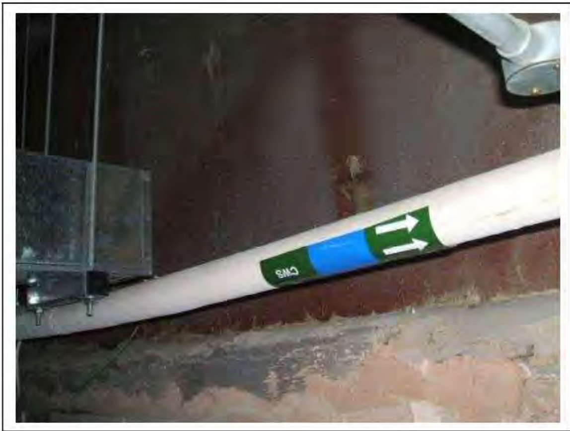
FIGURE 53: PRESUMED ASBESTOS IN RESIDUE IN FEMALE W/C, 2/416 - DESCRIPTION & RESULT OF ASSESSMENT (SAMPLE REF. P1&2(39))
