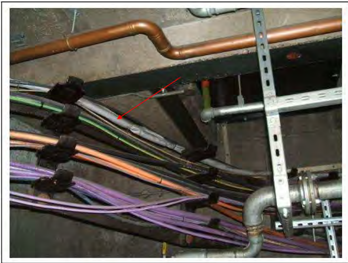
FIGURE 79: KNOWN ASBESTOS IN BRAIDED CABLES IN LMC, 3/161 - DESCRIPTION & RESULT OF ASSESSMENT (SAMPLE REF. K1(12))
