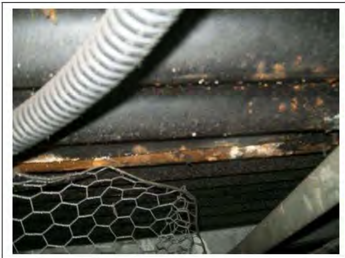
FIGURE 85: KNOWN ASBESTOS IN CELLACTITE IN PASSAGE , 3/202 - DESCRIPTION & RESULT OF ASSESSMENT (SAMPLE REF. K1(14))
