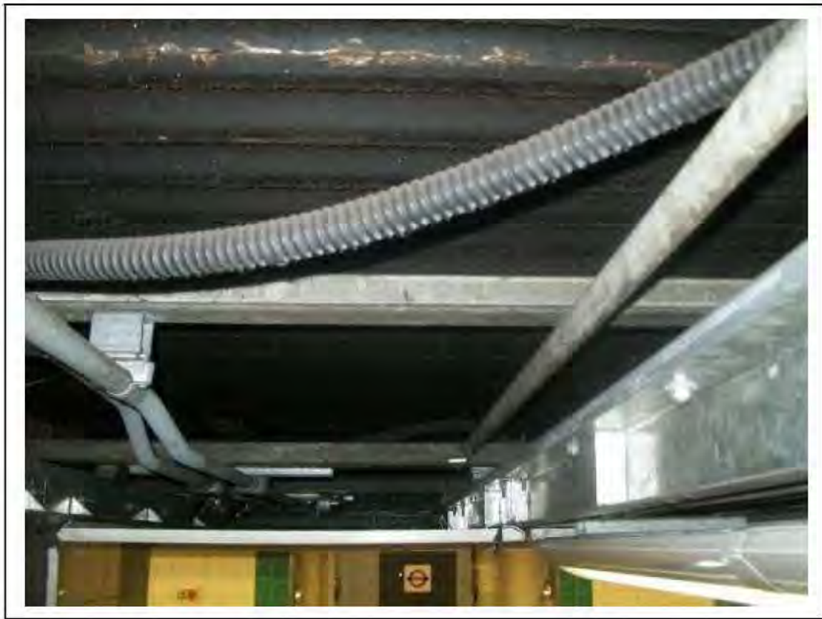
FIGURE 91: KNOWN ASBESTOS IN CELLACTITE IN PASSAGE, 3/205 - DESCRIPTION & RESULT OF ASSESSMENT (SAMPLE REF. K1(17))
