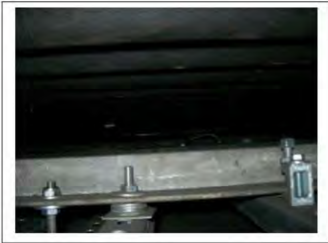
FIGURE 94: KNOWN ASBESTOS IN CELLACTITE IN PASSAGE , 3/207 - DESCRIPTION & RESULT OF ASSESSMENT (SAMPLE REF. K1(19))
