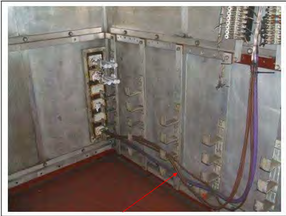
FIGURE 154: KNOWN ASBESTOS IN BRAIDED CABLES IN IMR, 3/706 - DESCRIPTION & RESULT OF ASSESSMENT (SAMPLE REF. K1(38))
