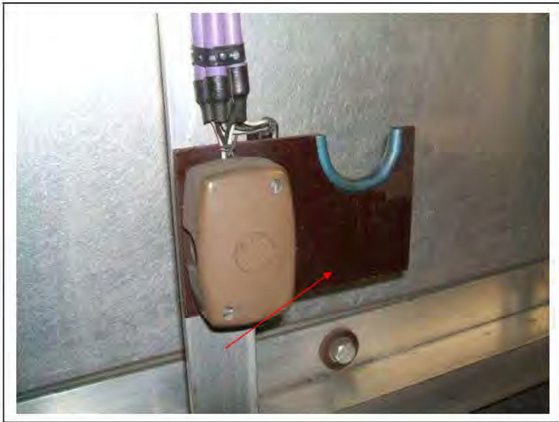
FIGURE 150: STRONGLY PRESUMED ASBESTOS IN SILUMINITE BOARD IN IMR (CORRIDOR FROM PLATFORM 1), 3/706 - DESCRIPTION & RESULT OF ASSESSMENT (SAMPLE REF. SP1(7))
