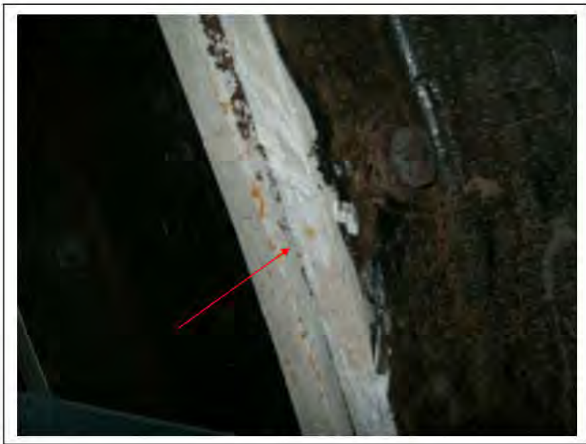
FIGURE 181: CONFIRMED ASBESTOS IN CAULKING IN OFFICE , 3/756 - DESCRIPTION & RESULT OF ASSESSMENT (SAMPLE REF. SAME AS 120445/150812/03)
