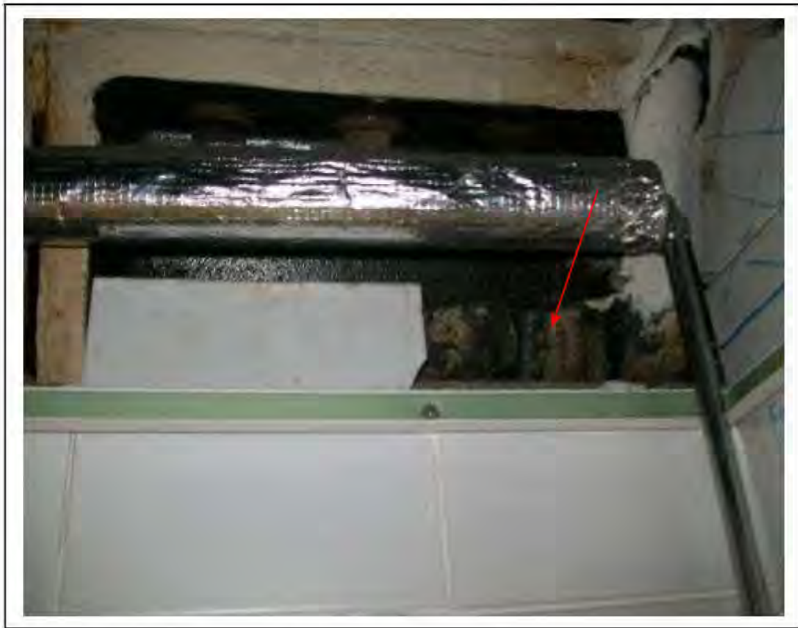
FIGURE 139: KNOWN ASBESTOS IN CELLACTITE CORRUGATED SHEETING IN LADIES W/C, 3/417 - DESCRIPTION & RESULT OF ASSESSMENT (SAMPLE REF. K1(34))
