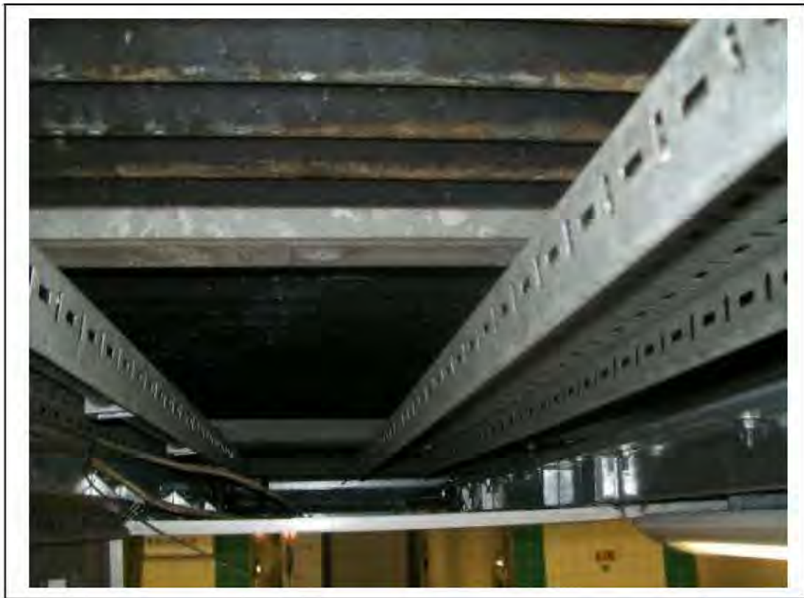
FIGURE 89: KNOWN ASBESTOS IN CELLACTITE IN PASSAGE , 3/204 - DESCRIPTION & RESULT OF ASSESSMENT (SAMPLE REF. K1(16))
