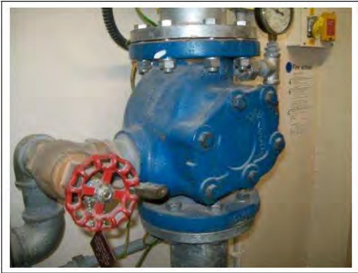
FIGURE 47: CONFIRMED ASBESTOS IN GASKET IN SVC, 2/401 - DESCRIPTION & RESULT OF ASSESSMENT (SAMPLE REF. 120445/160812/02)
