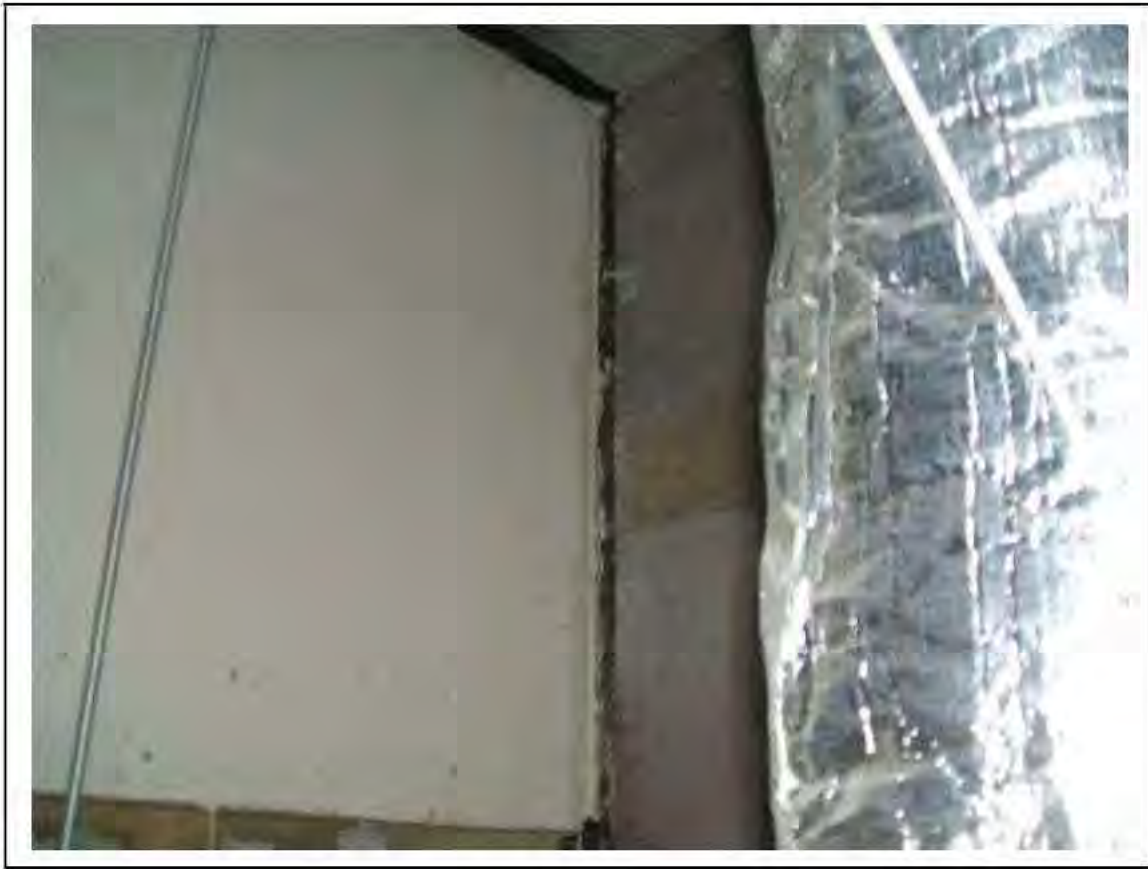
FIGURE 55: PRESUMED ASBESTOS IN RESIDUES IN MALE W/C, 2/417 - DESCRIPTION & RESULT OF ASSESSMENT (SAMPLE REF. P1&2(41))
