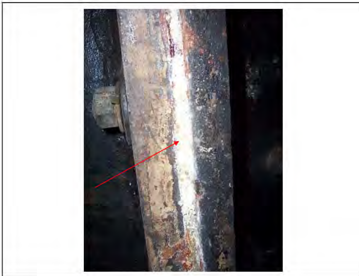
FIGURE 104: CONFIRMED ASBESTOS IN CAULKING IN PLATFORMS 1 & 2, 3/261 & 3/262 - DESCRIPTION & RESULT OF ASSESSMENT (SAMPLE REF. 061128/24SPH)
