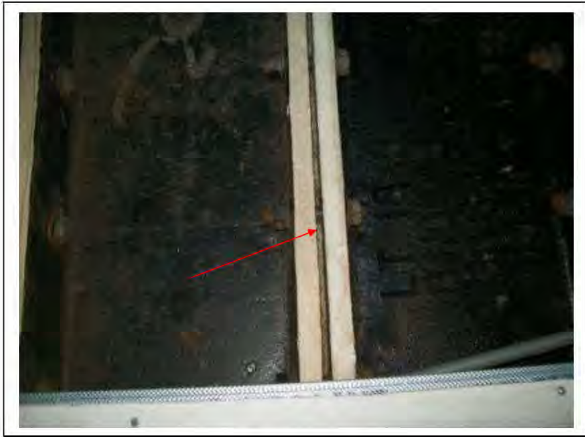
FIGURE 77: CONFIRMED ASBESTOS IN CAULKING IN MALE W/ C, 3/082 - DESCRIPTION & RESULT OF ASSESSMENT (SAMPLE REF. SAME AS 120445/150812/03)
