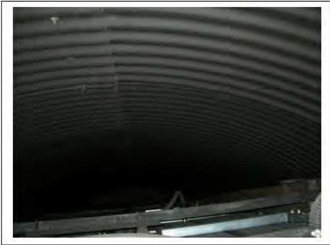
FIGURE 98: KNOWN ASBESTOS IN CELLACTITE IN PASSAGE , 3/208 - DESCRIPTION & RESULT OF ASSESSMENT (SAMPLE REF. K1(22))
