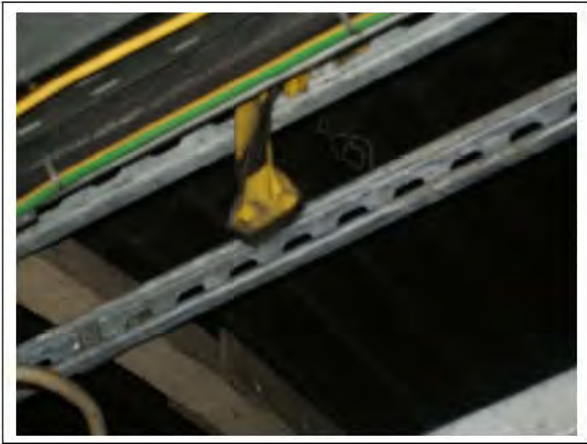
FIGURE 76: KNOWN ASBESTOS IN CELLACTITE IN LOWER CONCOURSE , 3/081 - DESCRIPTION & RESULT OF ASSESSMENT (SAMPLE REF. K1(10))
