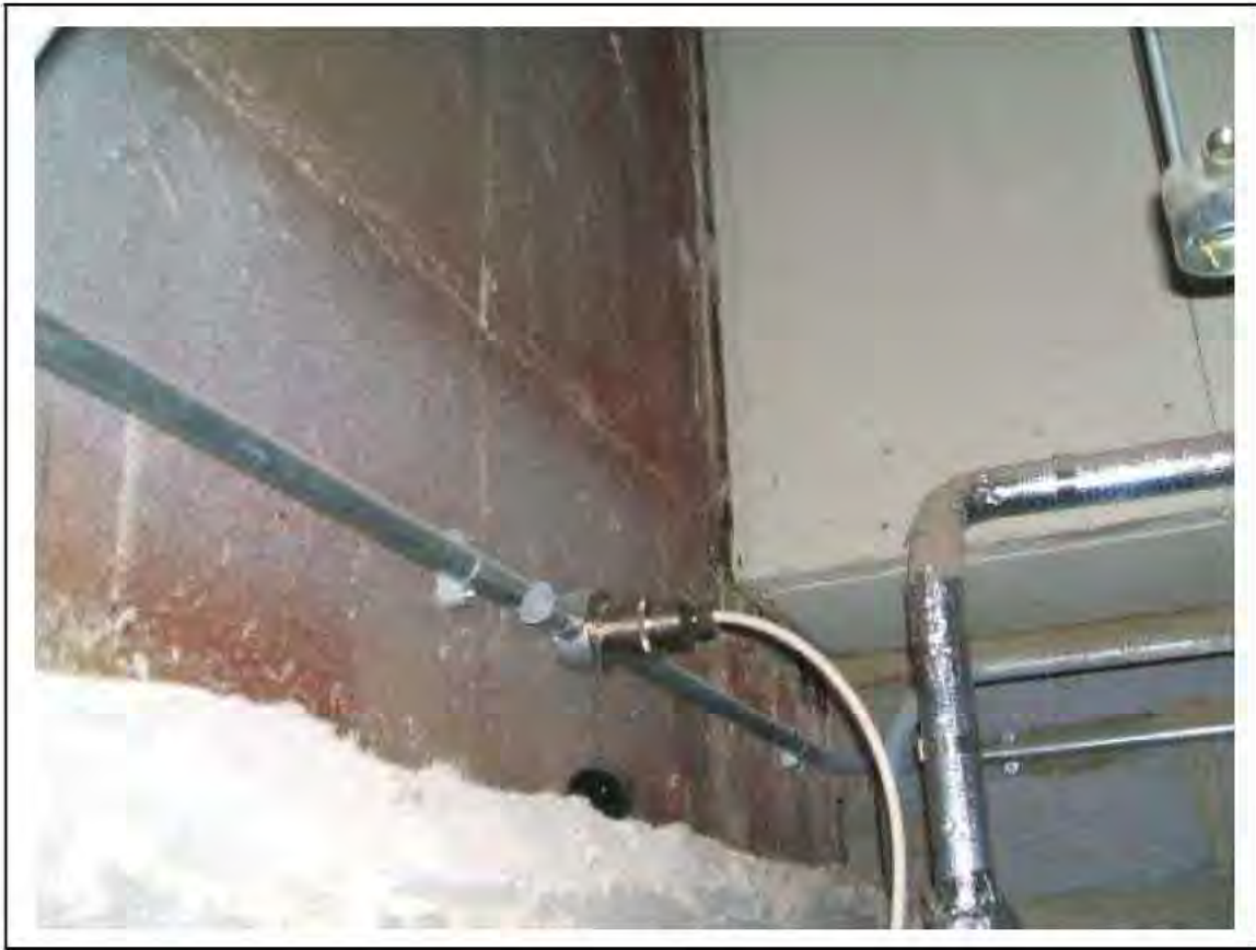
FIGURE 52: PRESUMED ASBESTOS IN RESIDUE IN FEMALE W/C, 2/416 - DESCRIPTION & RESULT OF ASSESSMENT (SAMPLE REF. P1&2(38))
