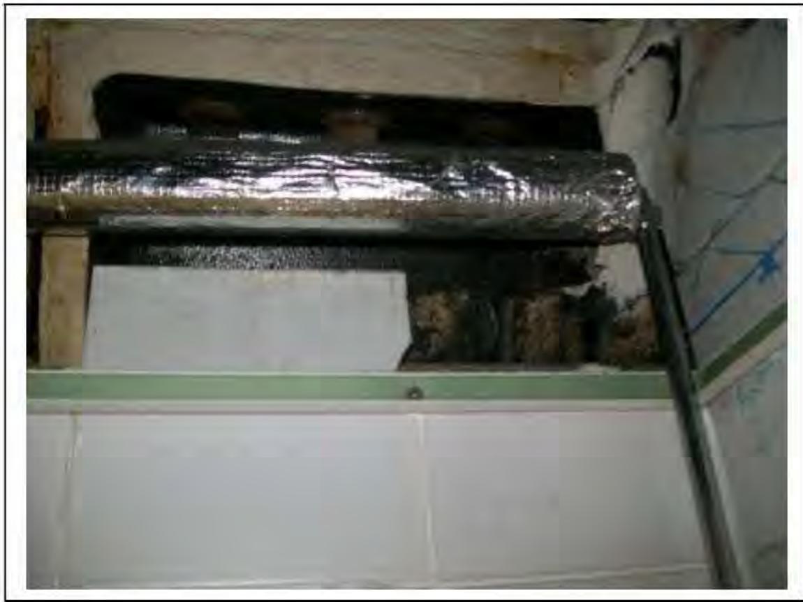
FIGURE 78: KNOWN ASBESTOS IN CELLACTITE CORRUGATED SHEETING IN MALE W/ C, 3/082 - DESCRIPTION & RESULT OF ASSESSMENT (SAMPLE REF. K1(11))
