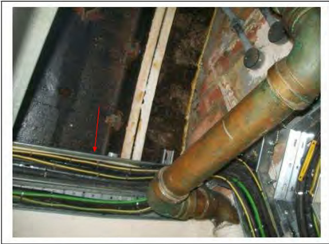
FIGURE 72: KNOWN ASBESTOS IN CELLACTITE IN SWITCH ROOM E14, 3/047 - DESCRIPTION & RESULT OF ASSESSMENT (SAMPLE REF. K1(8))
